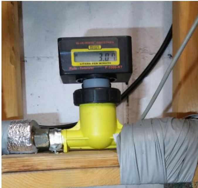
Figure 5. Flow meter for hot water flow measurement
