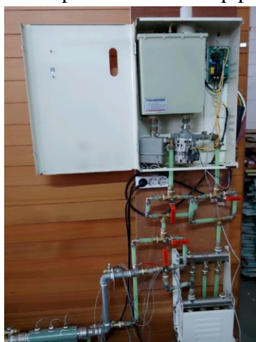
Figure 3. Hot water boiler that supplies thermal energy to the hot water circulating in the tubes in the hot water panels
