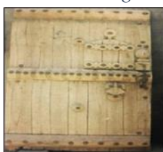
Figure (3) one-shutter door made of optimized wood
