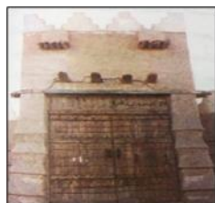
Figure 2 two-shutter big wooden door
